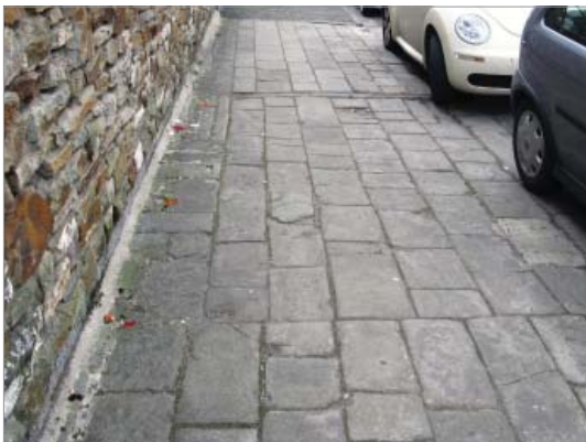
Stone paving in Richmond Road
