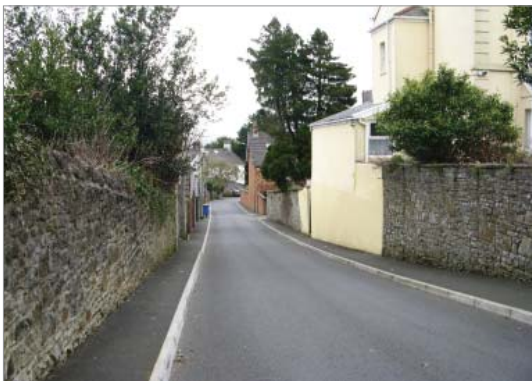
Stone walls in Belgrave Road
