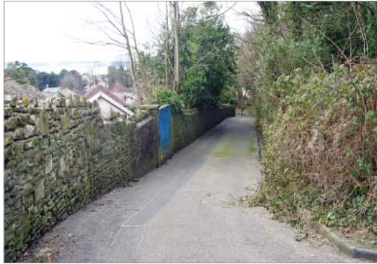
Stone walls in Terrace Road
