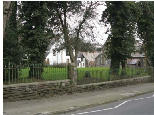
The listed railings around St James's Churchyard
